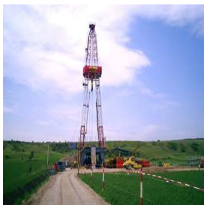
Forest Oil's exploratory rig in Romania
